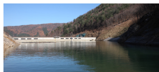
Water Supply Dam behind Valley Condo
